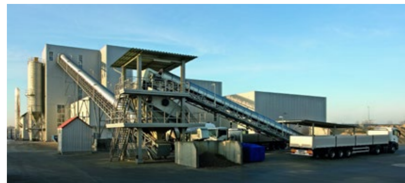
Sand is supplied and screened.
